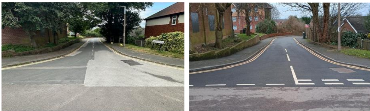
Figure 1 - Winlea Avenue Brecks, Before and After
