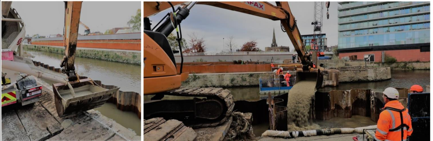
Figures 2 and 3 – De-watering the pouring points (behind the sheet piles) using an excavator (JCE, n.d.)
