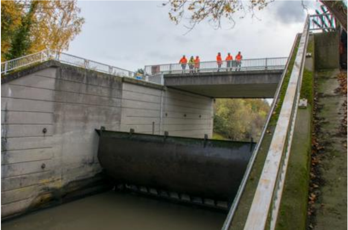
Meadowgate Flow Regulator - Previous Installation ('fish belly' gate)
