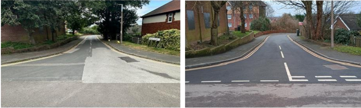
Figure 1 - Winlea Avenue Brecks, Before and After
