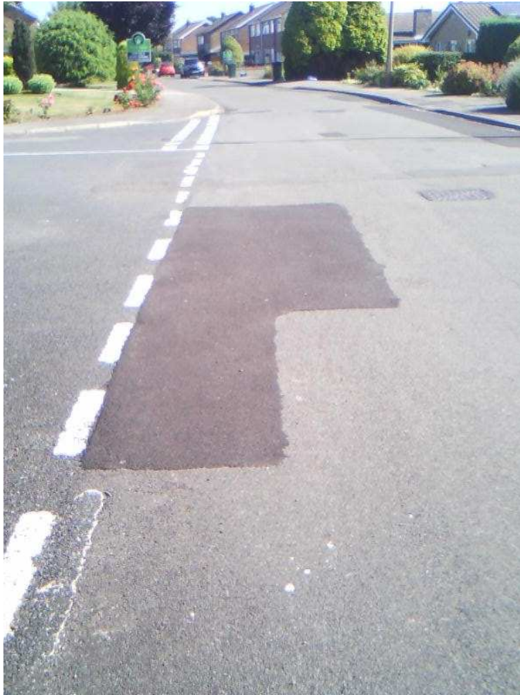
This shows the P5 patch has not deteriorated during the winter season.
