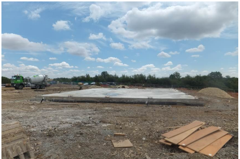
Reception building slab foundation complete.
