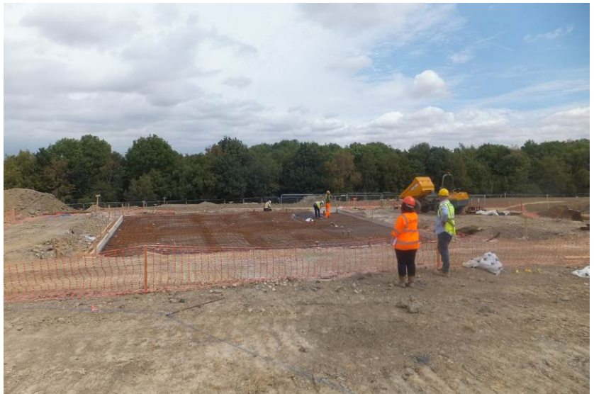
Reinforcing being positioned for the slab foundation, toilet block B.
