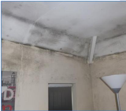
Picture 4: Black spot mould following condensation to walls and ceiling.
