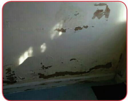
*Penetrating damp to internal wall with defective wall tiles to shower area at other side.*
