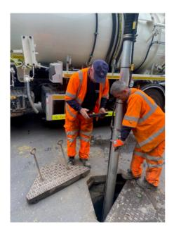
The gully cleansing schedule is now fully electronic, the team are collecting data on all gullies that are cleansed with information on:
