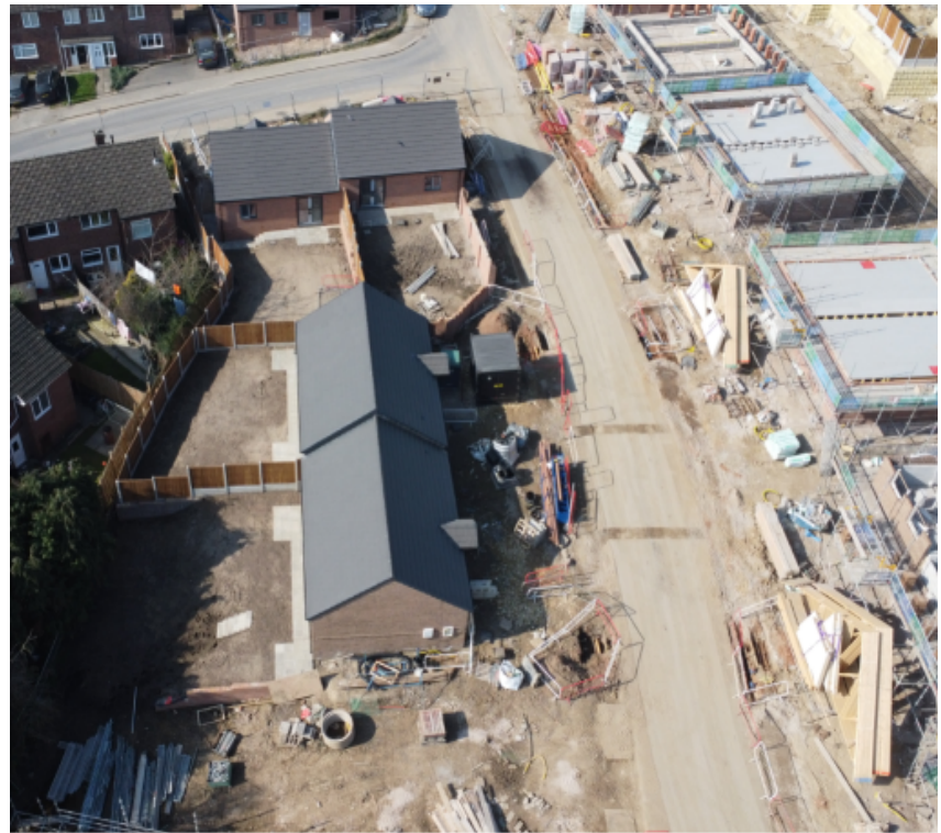
Image: The bungalows and apartments under development at Chesterhill.
