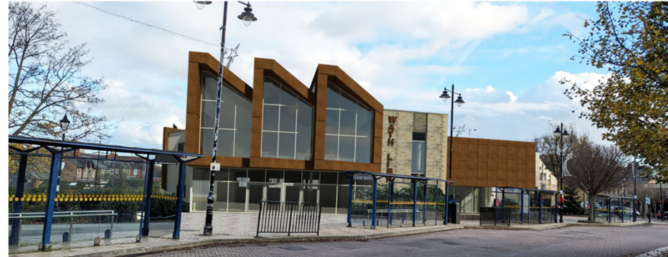
Western Facade from Montgomery Road
