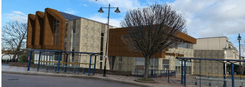
South and West Facades from Church Street
