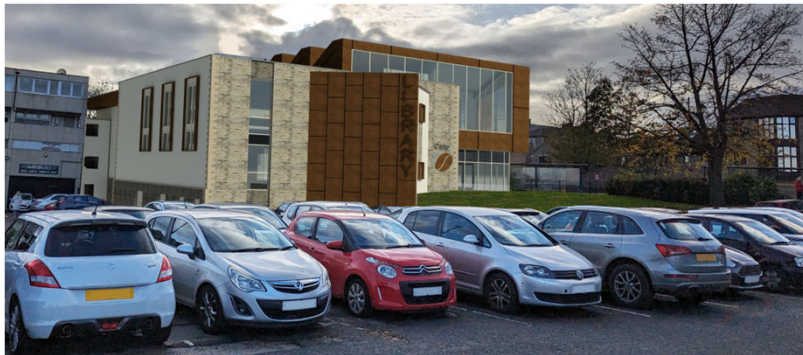
Northern Facades from Biscay Way
